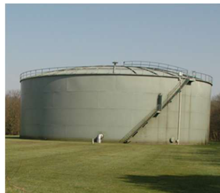
2 Renovatie rein waterreservoirs
